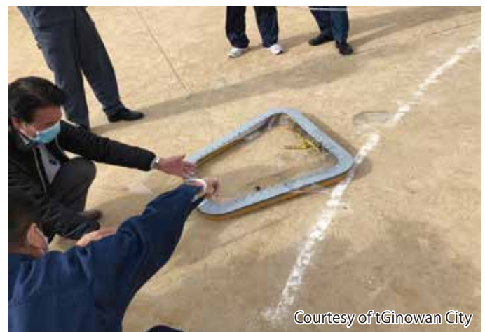
Ginowan City Futenma Daini Elementary School parts falling accident(2017)
