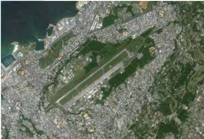
Figure: Aerial photograph of Futenma Air Base and location of schools
