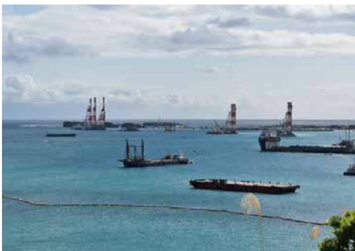
2025 70,000 piles need to be bored to reclaim land off Henoko
